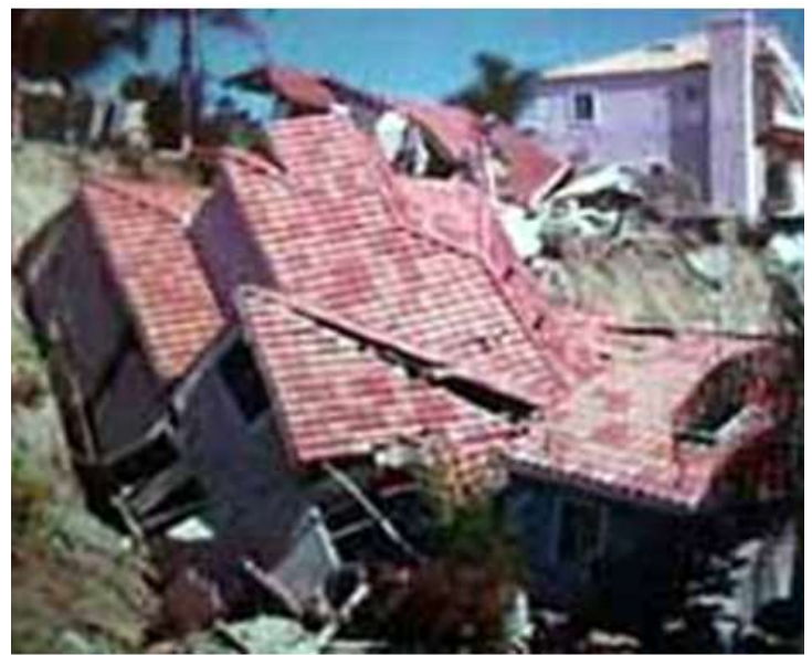
Figure 6: Laguna Nigel, California Landslide
