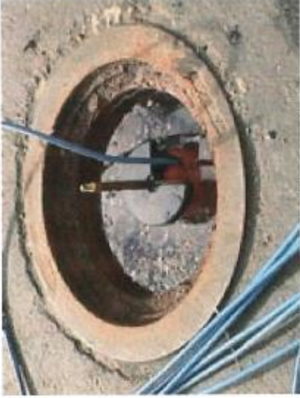
9. Using hanger to hold string during installation
