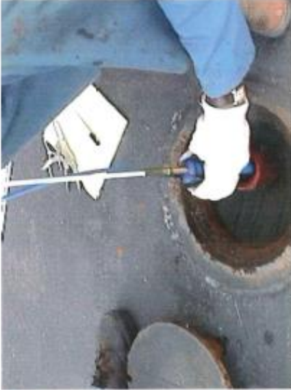
9. Lowering Little Dipper and rod assembly
