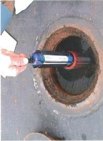
8. Aligning guide fins with casing grooves
