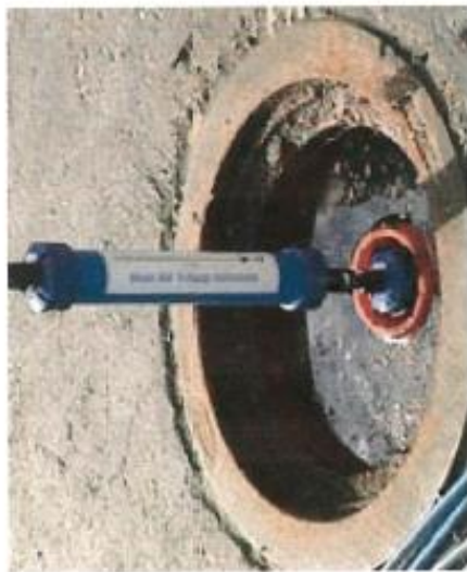
7. Universal pivot inserted into casing grooves - ready for lowering
