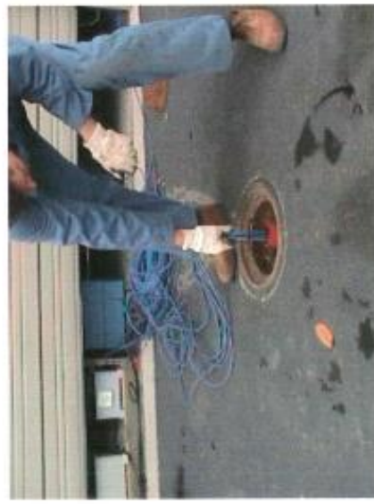
16. The string is pushed into the hole for the length of the push/pull rod...
