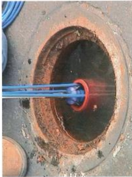
13. Multiple cables led up between guide fins on Little Dipper
