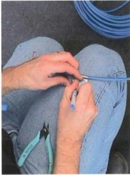
2. Labeling cable end
