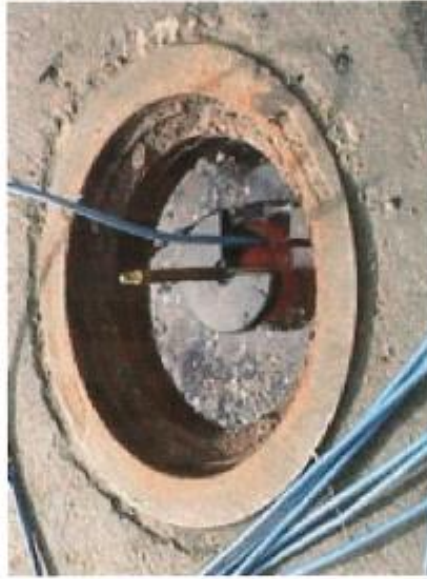
11. Using hanger to suspend string during Little Dipper installation
