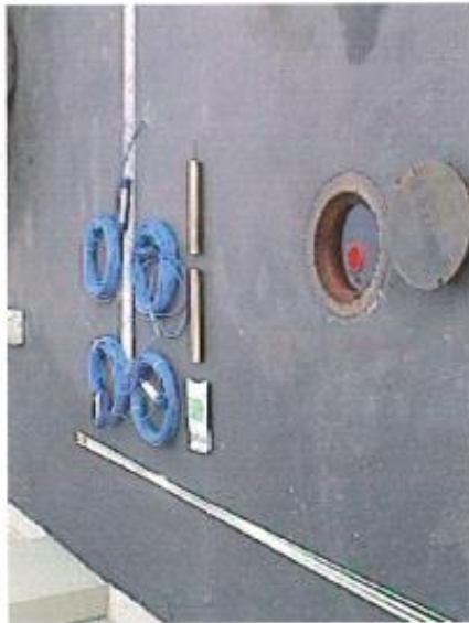
1. Equipment ready for installation
