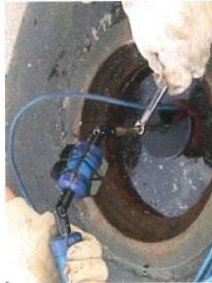
10. Attaching connecting rod to next universal pivot (Little Dipper attached) using 7/16 open end wrench
