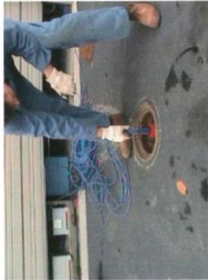
13. The string is pushed into the hole for the length of the push/pull rod
